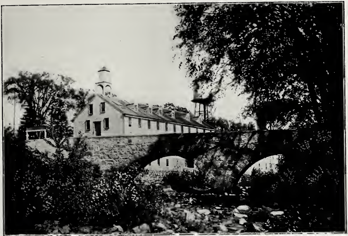
ARCH BRIDGE, SHOWING SLATERSVILLE MILL, SLATERSVILLE
